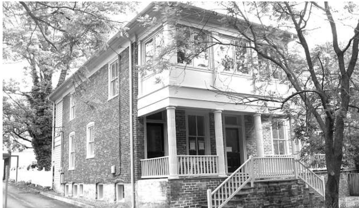
One of the two historical Musselman buildings now for lease on 7th Street
